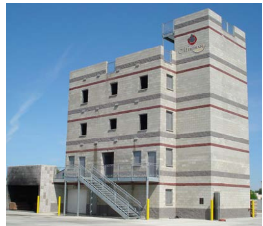
5-Story Training Tower 540 E Franklin Rd
